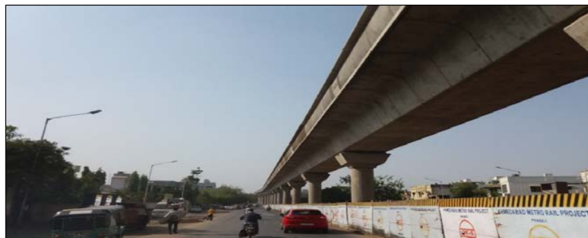
Fig 13 Viaduct construction work APMC to Shreyas
