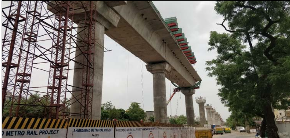
Fig. 14 Viaduct Construction work Shreyas to Ranip
