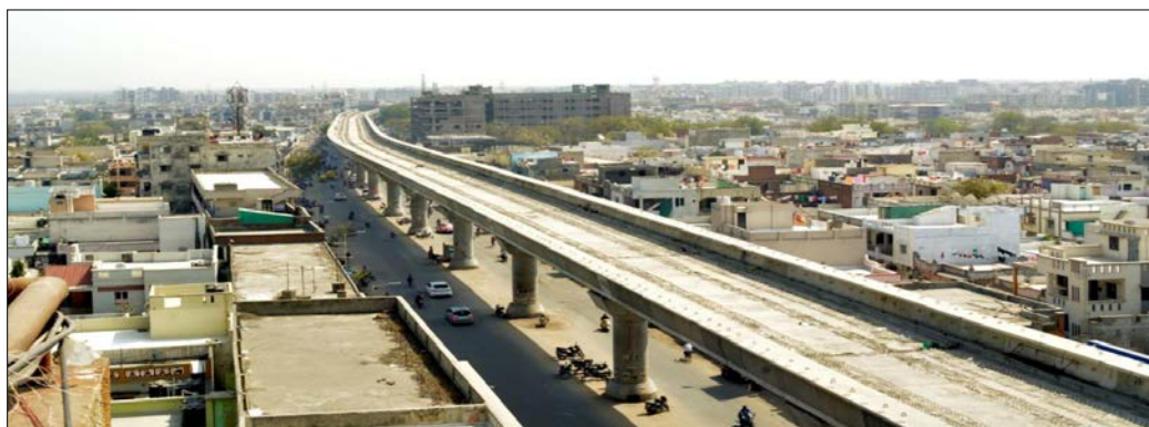
Fig. 1 Viaduct work from Vastral Gam to Apparel Park
