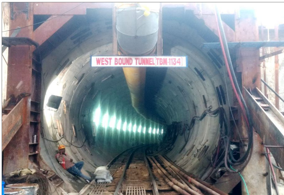
Fig. 7 TBM West bound Tunneling Work
