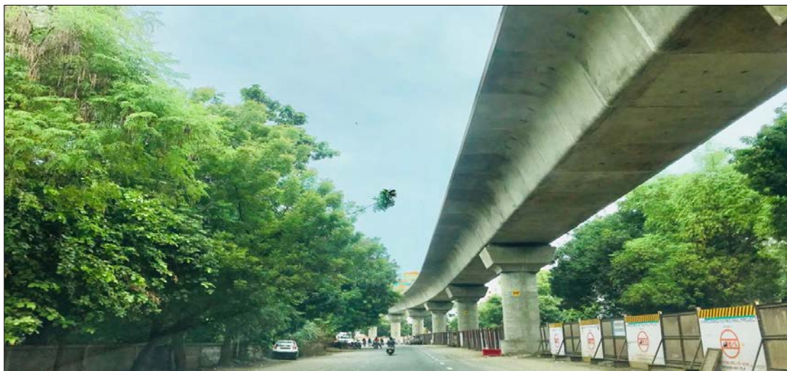
Fig. 3 Viaduct work - Thaltej to Stadium
