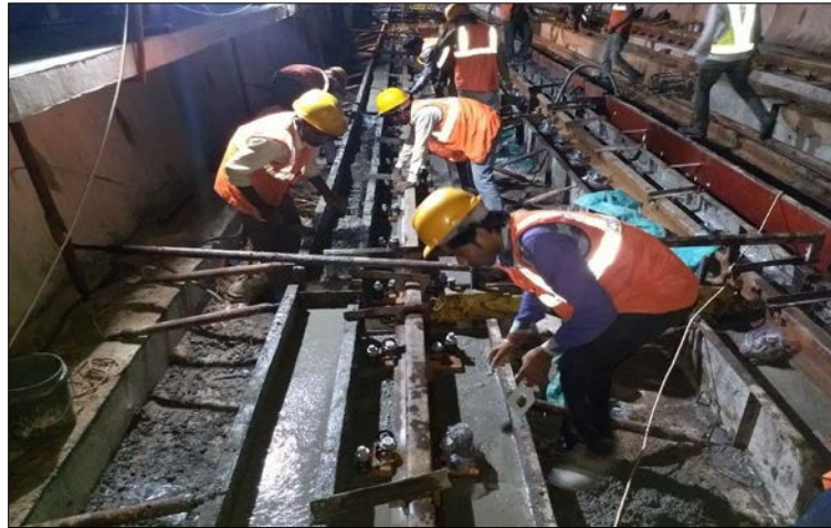
Fig. 2 Track laying work from Vastral Gam to Apparel Park
