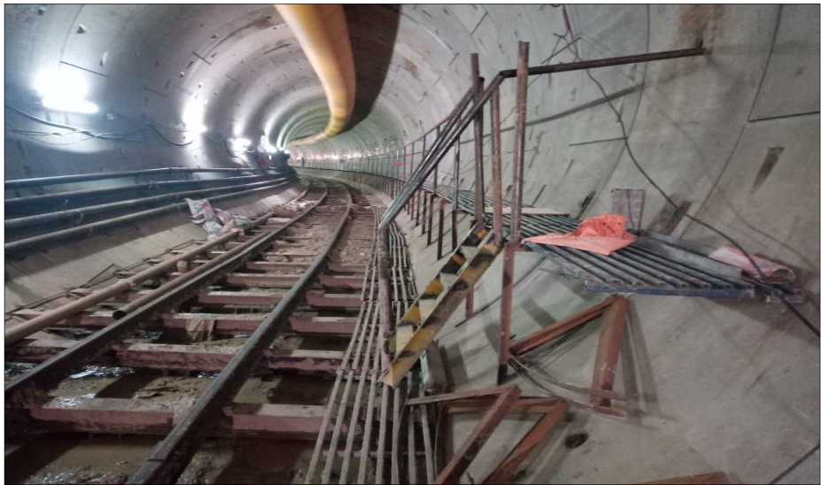
Fig. 6 Tunneling Work from Apparel Park to Kalupur
