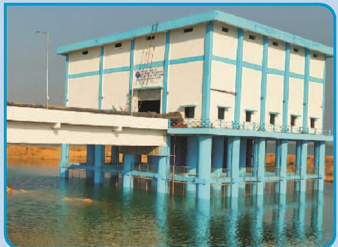
Brahmani 2 Dam Intake
