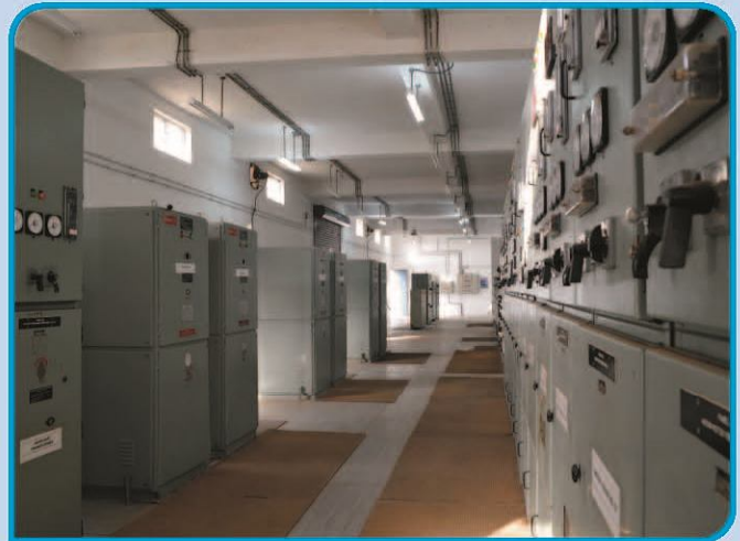
Anjar Pumping Station
