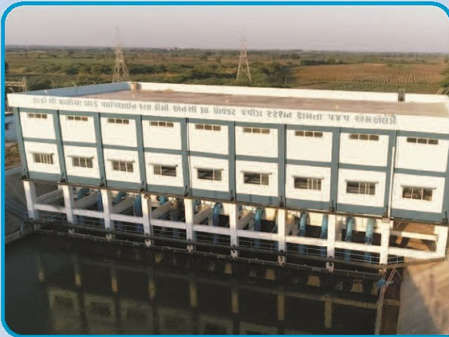
Dhanki Pumping Station NC-30 Project, Surendranagar
