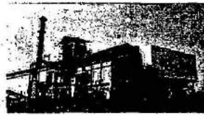
6.5 MW Power Plant Mahabubnagar, AP
